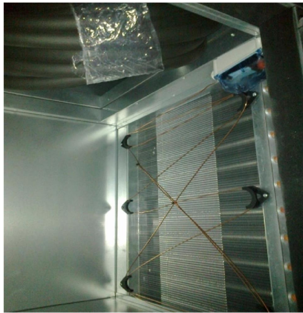
Figure 24 Ě Installation of capillary tube of TS1-C0P anti-freezing thermostat
