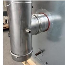
Figure10 Placement of sump for flue gas
