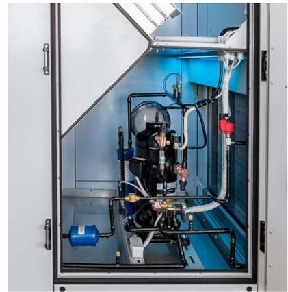
The units may be designed with the primary recuperation section (plate/rotary exchanger air/air) or the refrigerant circuit as a separate element in the supply-discharge unit. The unit may be additionally fitted with a bivalent heat source – additional water/electrical/gas heating.
